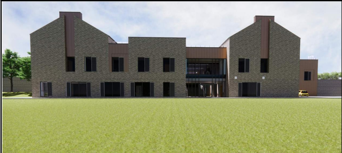
Figure 4 – Rear view from Bedwellty Park (looking westwards)
